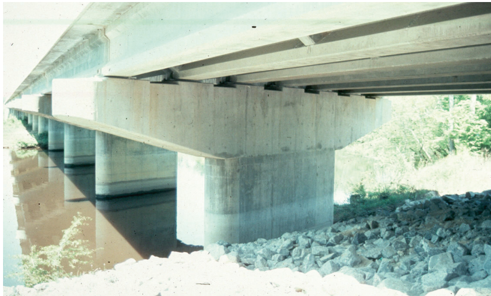
Figure 11.3.19 Cantilever or Hammerhead Pier
