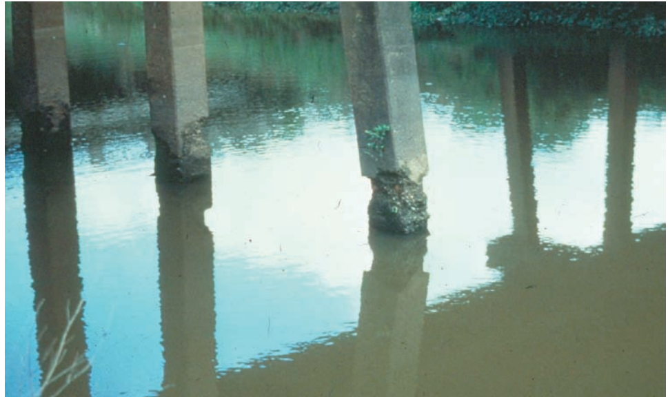
Figure 11.3.26 Concrete Deterioration
