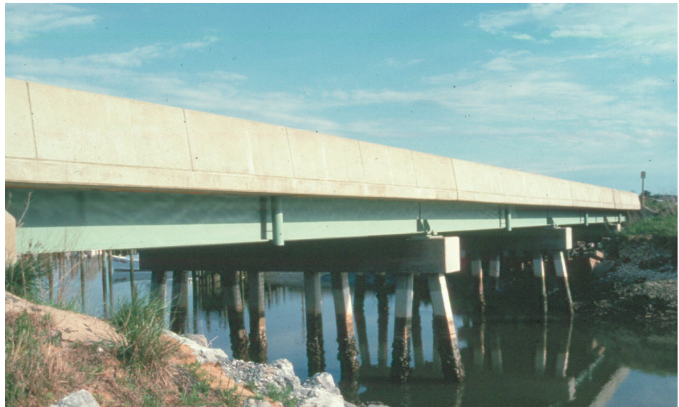
Figure 11.3.17 Concrete Pile Bent
