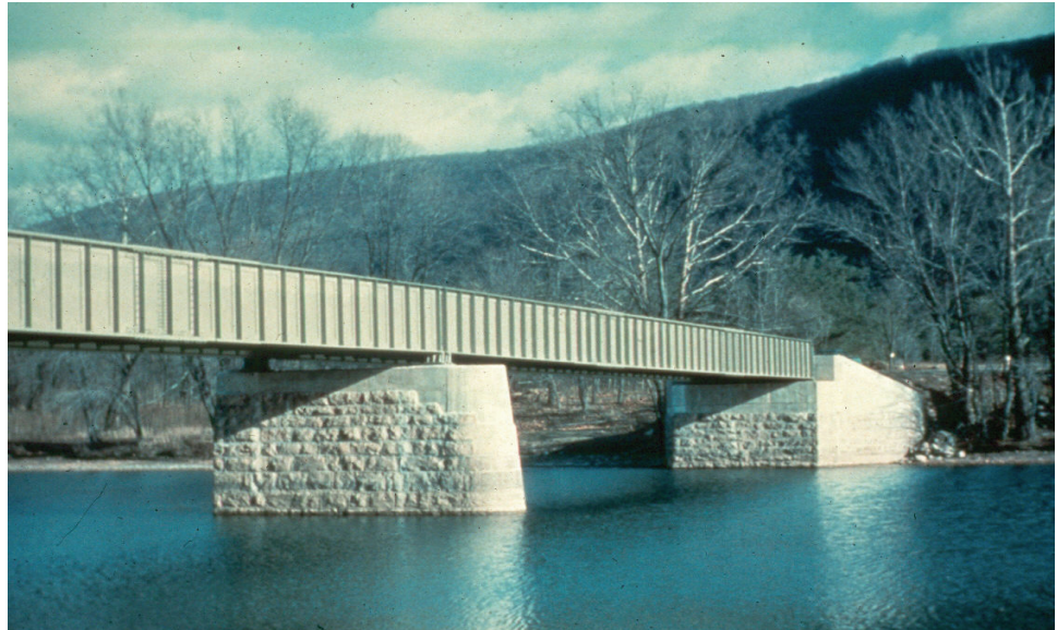
Figure 11.3.20 Solid Shaft Pier
