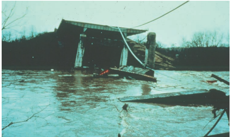
Figure 11.3.1 Schoharie Creek Bridge Failure
