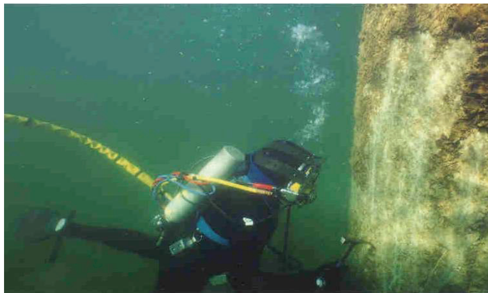
Figure 11.3.6 Diver Cleaning Pier Face For Inspection
