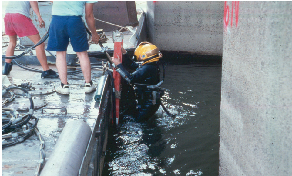
Figure 11.3.38 Access Barge and Exit Ladder
