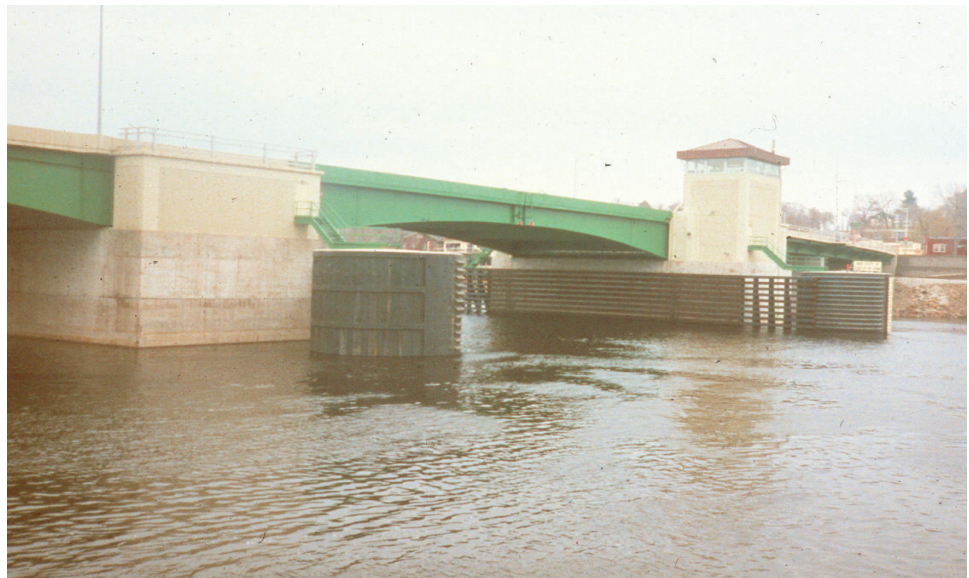
Figure 11.3.7 Bascule Bridge on the Saint Croix River
