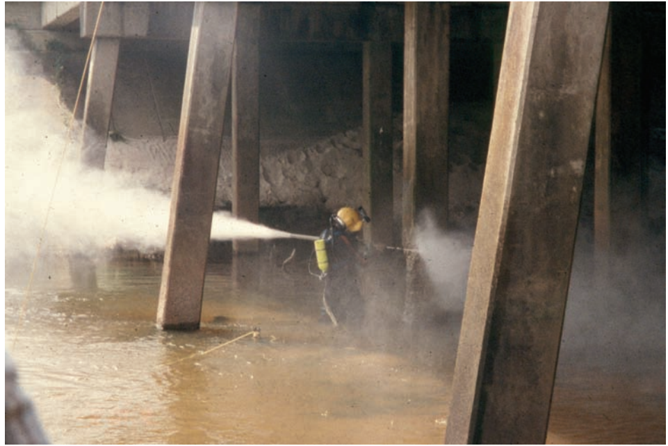
Figure 11.3.41 Cleaning with a Water Blaster
