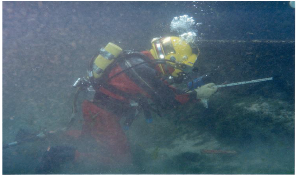
Figure 11.3.5 Surface-Supplied Diving Inspection
