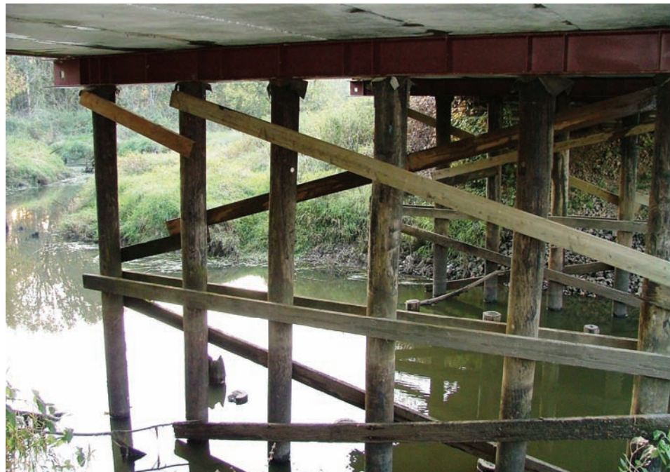
Figure 11.3.15 Timber Pile Bent
